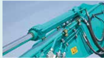
Dismantling bucket cylinder
